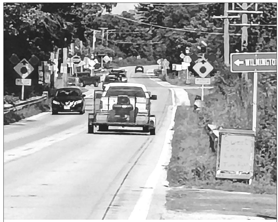
A NEW FOUR-WAY stop has been installed at the intersection of Route 113 and West River Road to reduce the number of accidents in the area.
