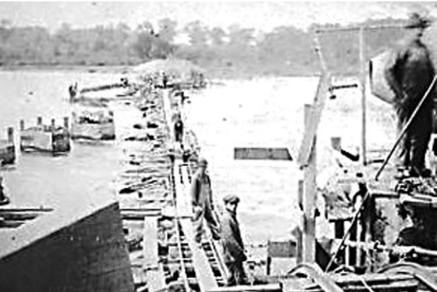
A PHOTO THE the dam under construction, paid for mostly by the paper company who needed the water higher in the mill race.
