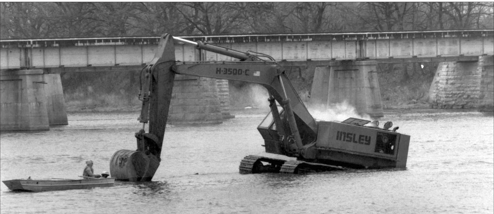
Free Press file photo CREEPING ACROSS THE Kankakee River a mile upstream of the Grundy-Will County line is a Insley crawler excavator used in 1987 to bury three 30-inch pipes for the Dresden warm water discharge. The Army Corps of Engineers' project was behind schedule by three weeks due to equipment failures, piping delays and extremely cold days.
