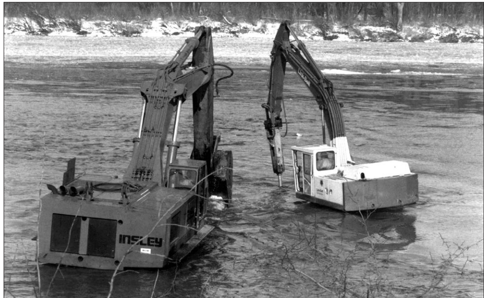
Free Press file photo IT WAS 38 YEARS ago when the U.S. Army Corps of Engineers hired workers to install the warm water discharge pipes in the Kankakee River near Cottage Road. The $400,000 project included the installation of three 30-inch pipes, 200 feet apart, across the length of the river.
