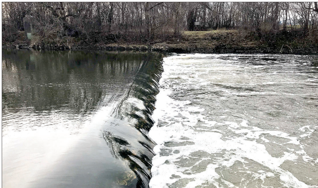
THE LOWHEAD DAM at Hammel Woods will be removed under safety concerns by the Will County Forest Preserve.
