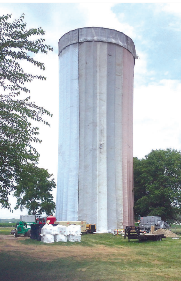
AT ONE POINT the village water tower at North Park looked more like a grain silo than a water reservoir. It was draped during restoration to allow for sand blasting and painting. Work started in early June and completed last week.
