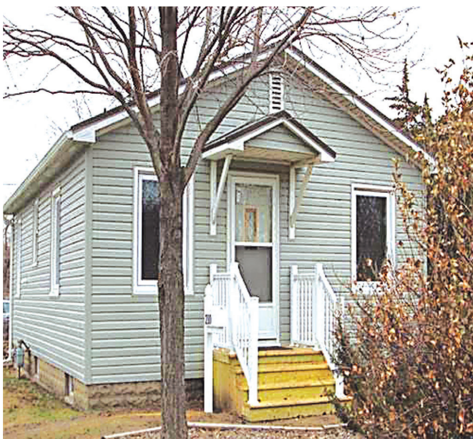
IMPROVEMENT PROJECTS for 25 homeowners in Coal City included energy saving windows, siding and doors. Interior repairs included flooring, electrical upgrades, plumbing and HVAC systems.
