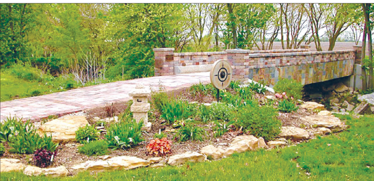
JAMES KRAFT'S BRIDGE that incorporates many of his antique bricks.
