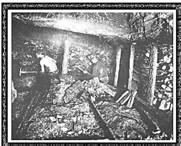
A TYPICAL "ROOM" in a shaft mine, taken in 1912 at the "G" shaft mine.
