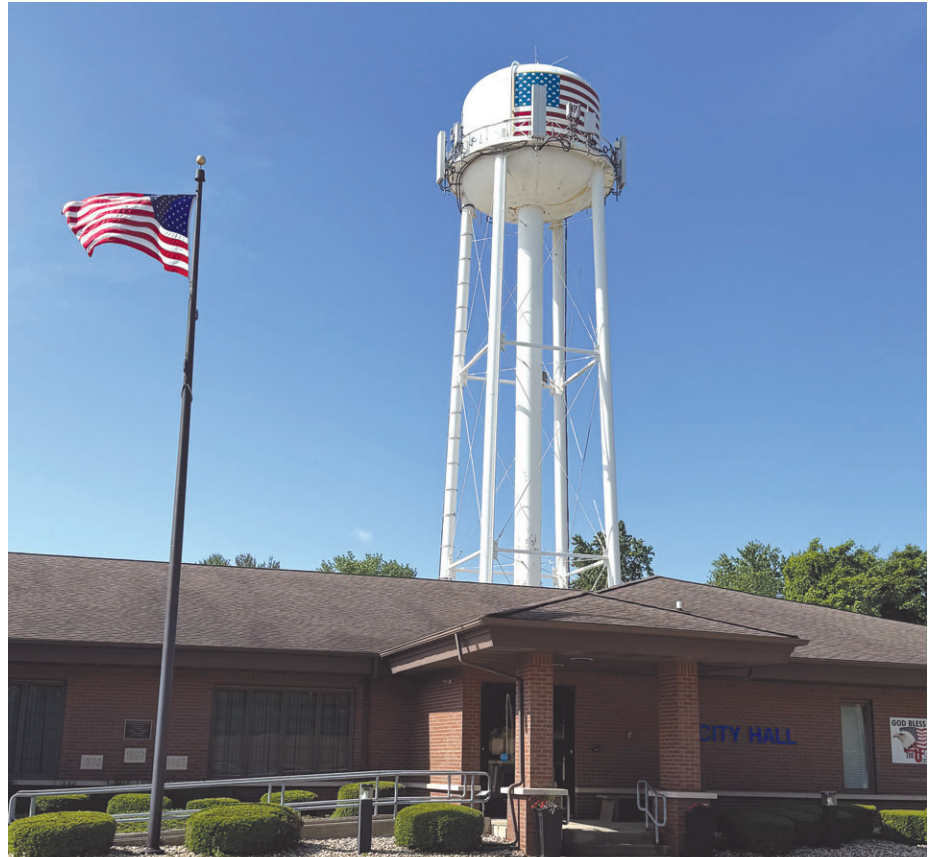
THE MAIN STREET water tower behind the Braidwood City Hall is operational again after undergoing repairs. The town was non-operational since late November.
