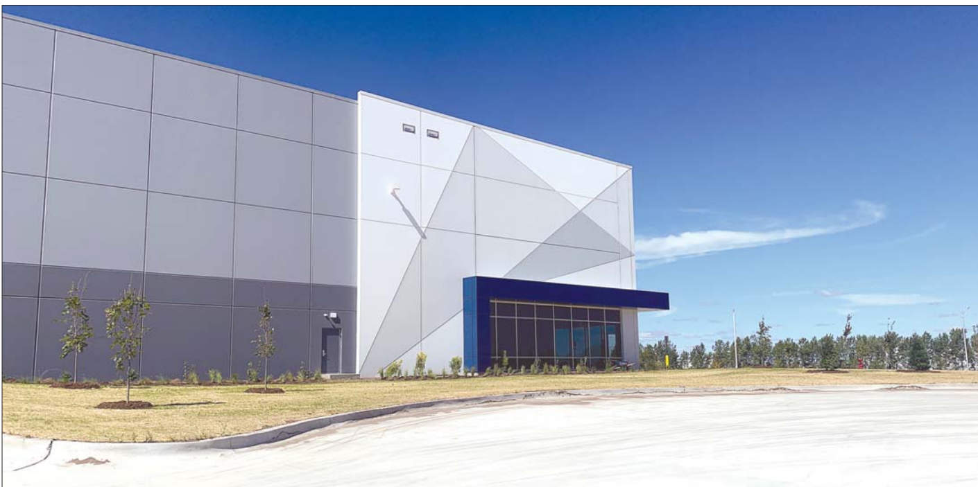
WOLF HOME PRODUCTS has occupied a 1 million-plus sq. foot warehouse at 30350 S. Graaskamp Blvd, Wilmington. It will be the largest warehouse for the York, PA company, serving nine states in the Midwest. The warehouse is expected to be fully operational at the end of the year.
