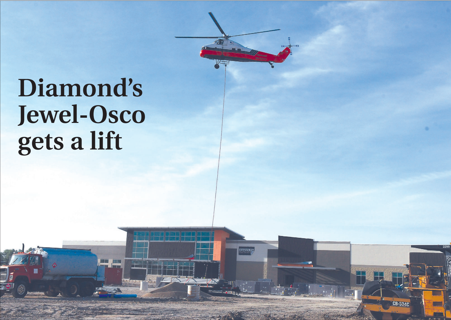
A SIKORSKY HELICOPTER operated by Midwest Helicopter Airways of Willowbrook lifts one of 19 refrigeration units for the new Jewel-Osco store being built in Diamond. Midwest Helicopter Airways lifted over 58,000 pounds of equipment onto the roof on Friday for contractor WA Randolph Company.
