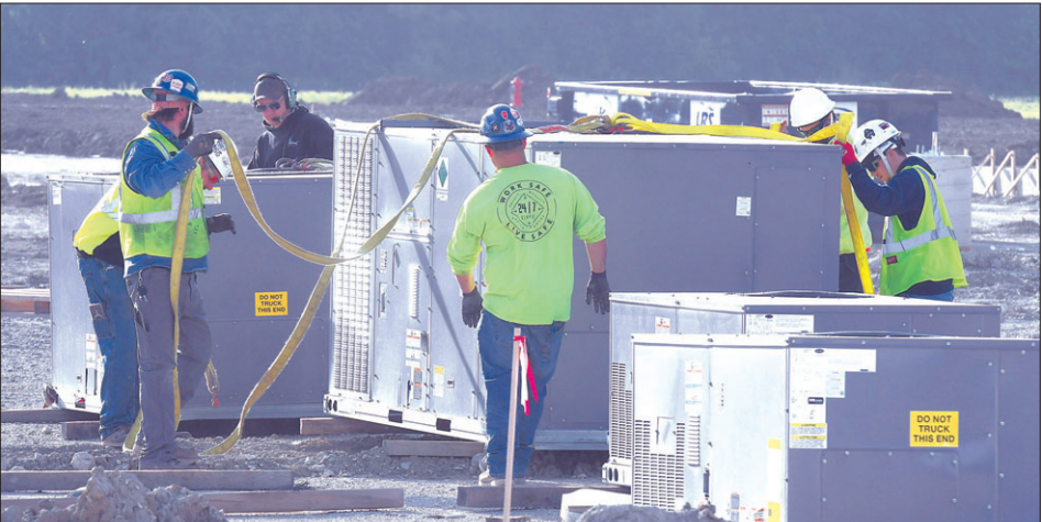
THE GROUND CREW—How do you lift a two ton cooling unit? With a skilled ground crew from WA Randolph Company of Gurnee, the contractor building the new Jewel Osco store in Diamond. Workers hustle to strap down the next lift as the helicopter drops the first unit onto the roof on Friday.
